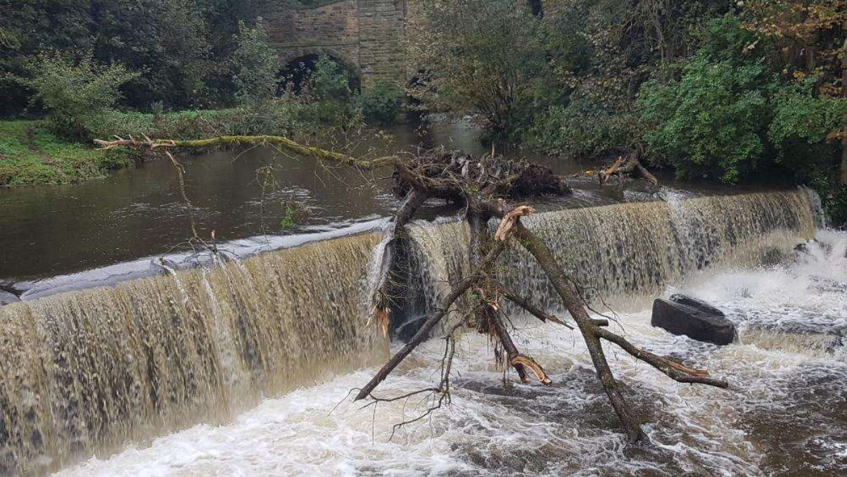
Large tree brought down by one of the storms rests atop the weir for several months
