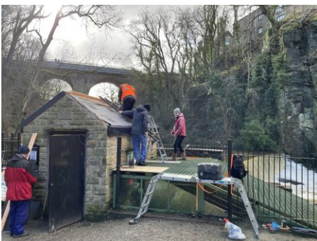
Opening up the roof
