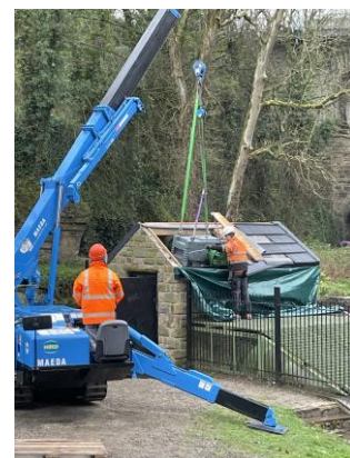
The gearbox being craned back into position
