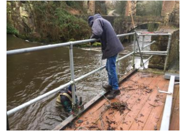
Routine clearing operations
